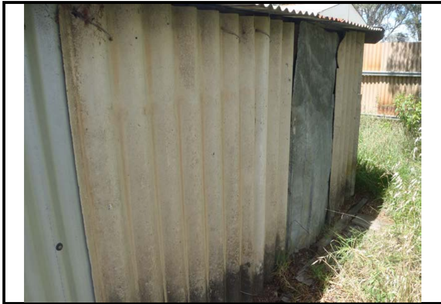
Photo 13: 14 Horton Road: A section of the corrugated ACM sheeting used to the exterior of the garage.
