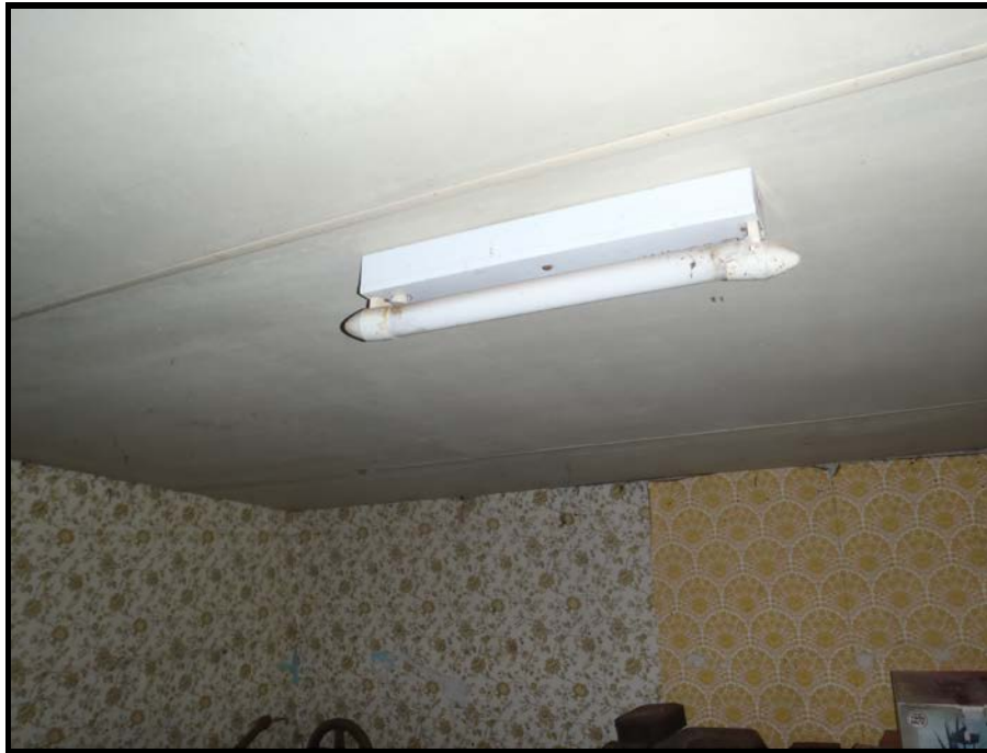
Photo 9: 14 Horton Road: An example of one of the fluorescent lights in the garage that may have a PCB-containing capacitor
