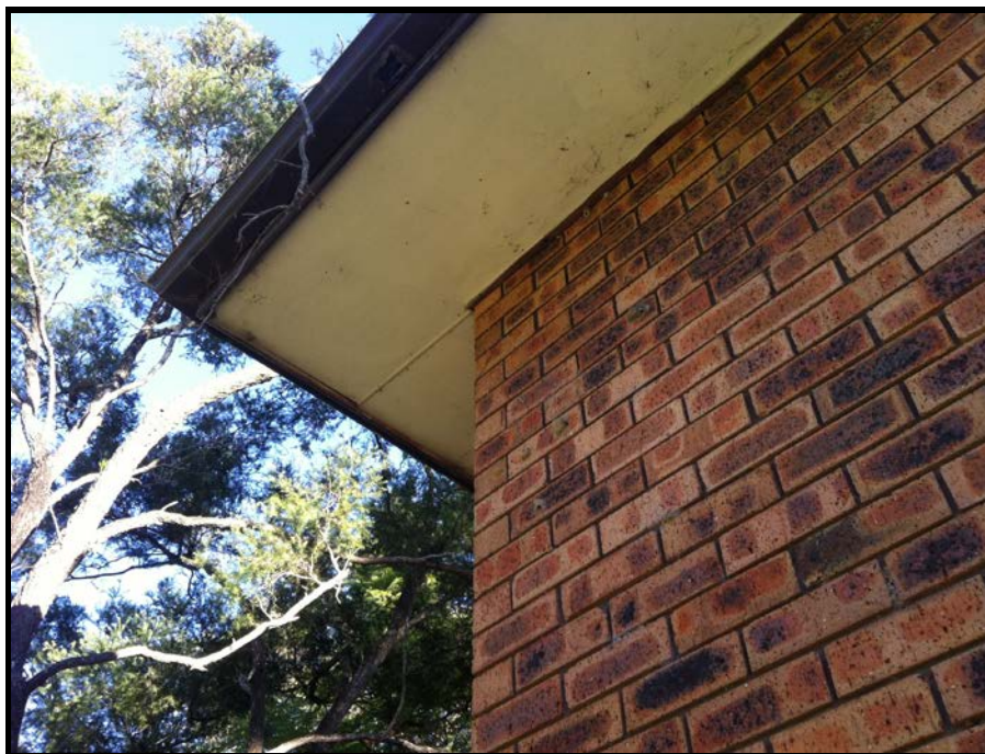
Photo 20: Scales Avenue: A section of the eaves lined with ACM sheeting.
