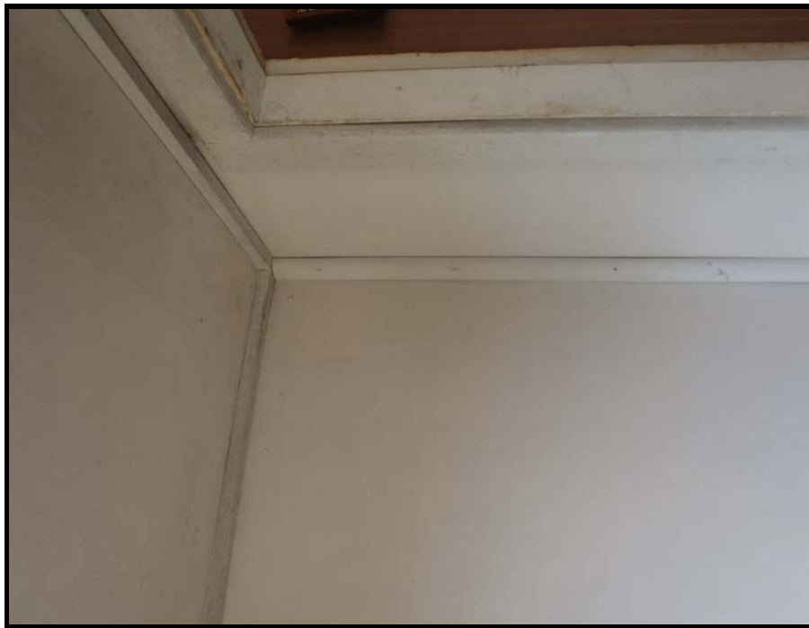
Photo 1: 14 Horton Road - Section of the ACM sheeting used in the walls and ceiling to the front door landing
