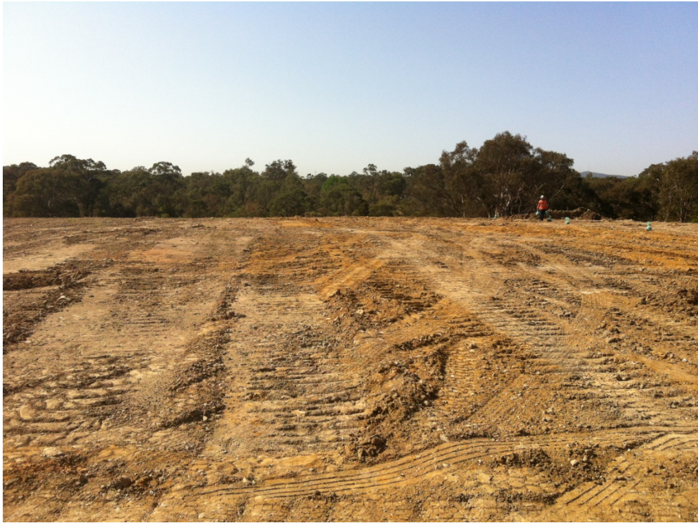
PHOTOGRAPH 1 Stockpile Surface (taken facing south-west)
