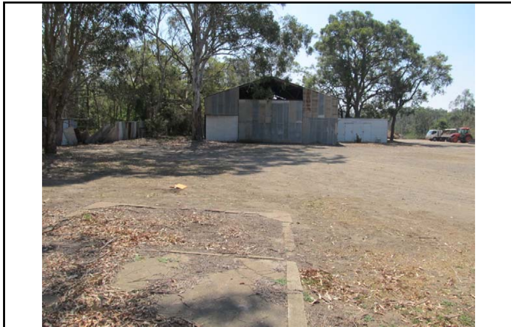
Photo 12: Photograph of front of Lot 16 looking north-west from Horton Road – ACM fragments found on exposed soil area in foreground.
