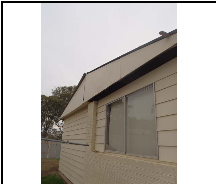
Photo 15: 12 Horton Road (residence): ACM sheet panels used to the exterior walls.
