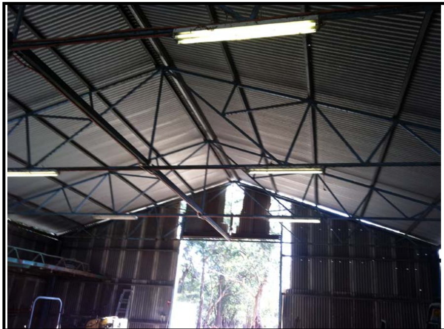
Photo 24: 12 Horton Road (Business): Fluorescent lights fitted to metal frame in large shed
