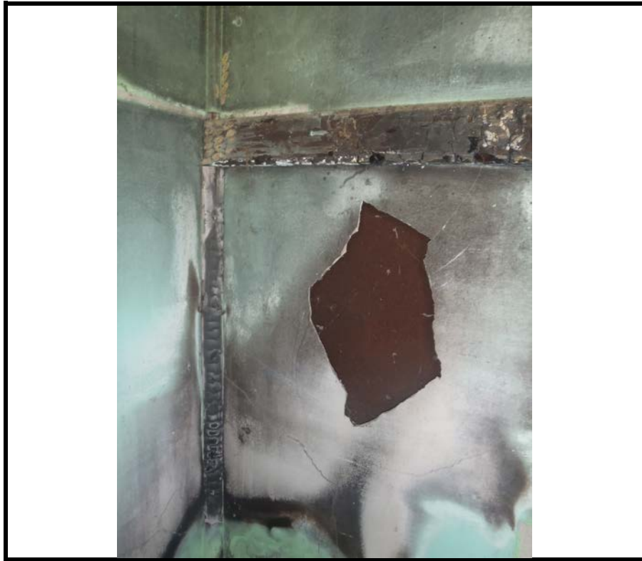
Photo 5: 14 Horton Road: An example of the damaged ACM sheeting within the laundry
