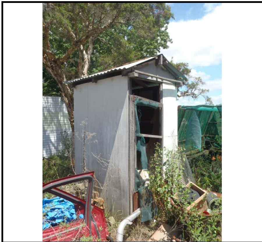
Photo 14: 14 Horton Road: The former outhouse with walls and gable ends lined with ACM sheeting.
