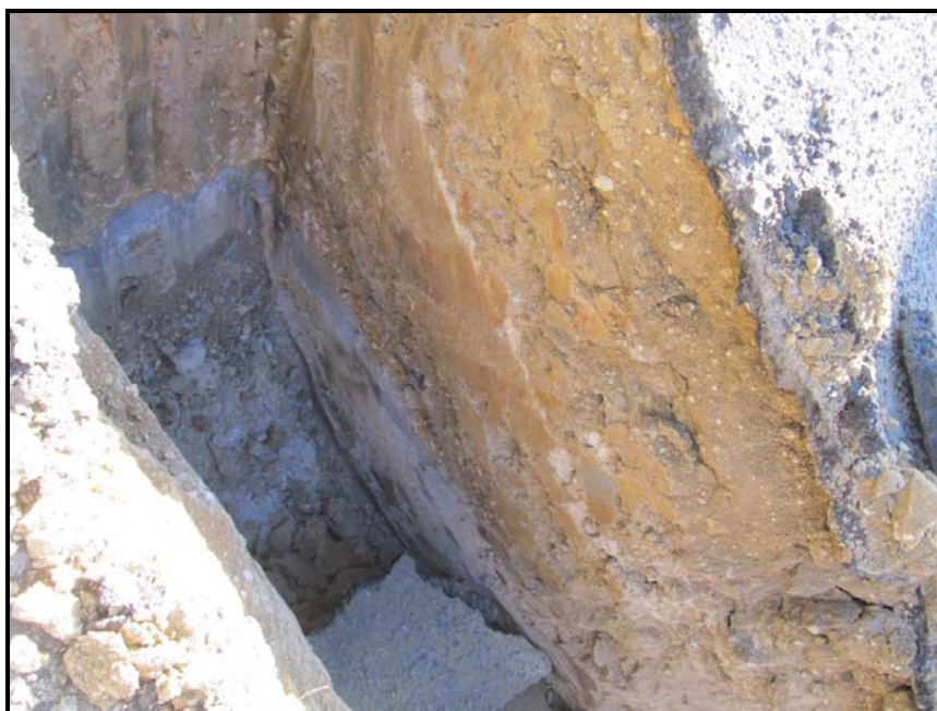
Photo 7: Photograph of clayey fill profile under carpark on Lot 420 .
